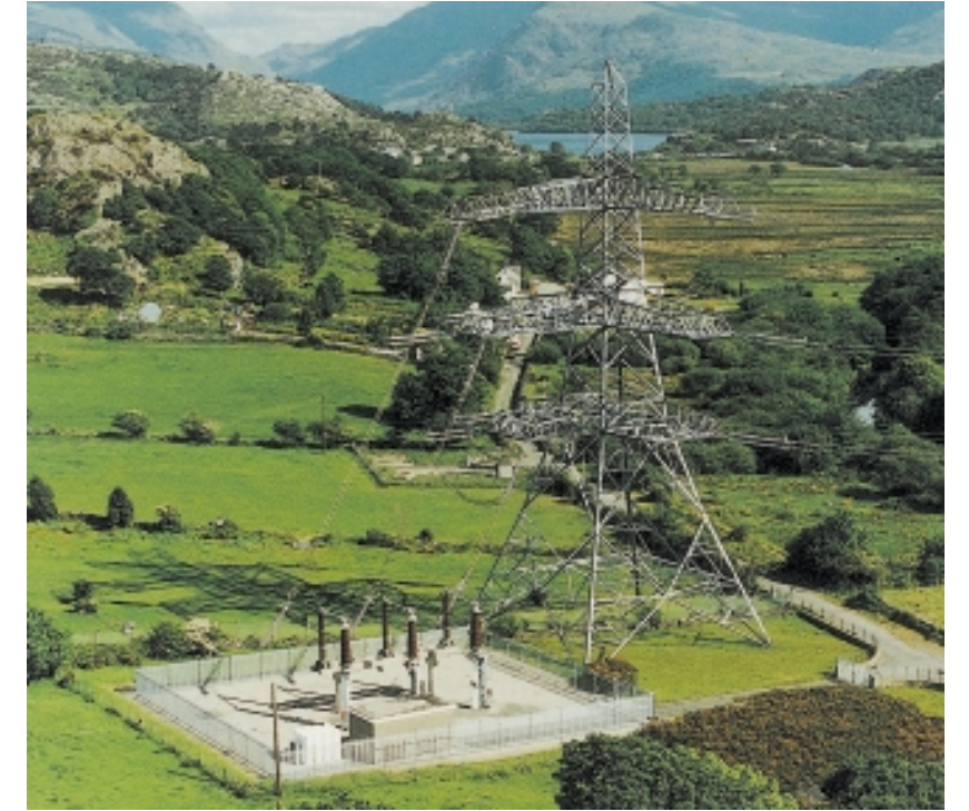
Jordkabels terminalstation
